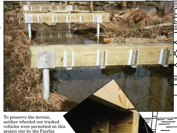
For elevation changes, the screw foundation shaft "reveal" above grade was varied within plan range.
